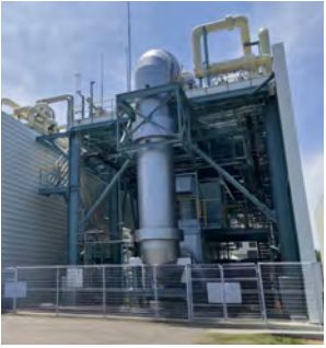
Cogeneration system compatible with hydrogen co-firing launched at our Yokohama Isogo Complex
